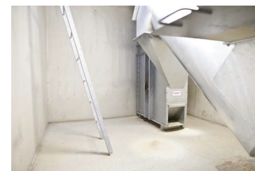
In de kelder
